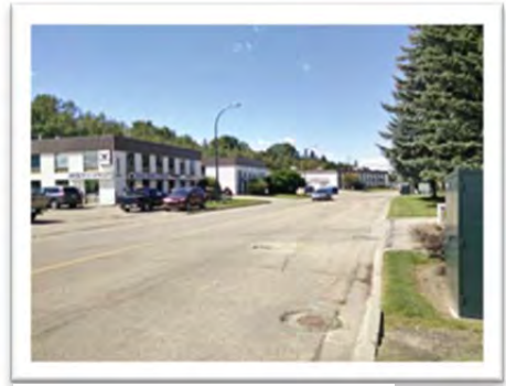
Missing sidewalks along 45 St
