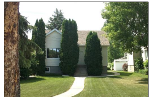
Minimal Traditional Style – renovated with vinyl siding
