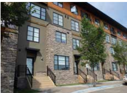
Apartment style building with street access.
