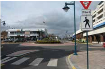
Highlight cross-walk at roundabout.
