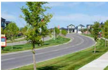
Example of separated sidewalk.
