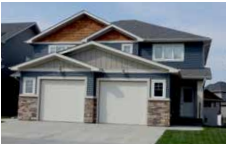
Semi-detached housing with front garage.
