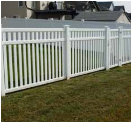
Continuous fencing along public areas.
