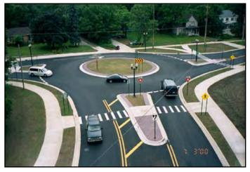
An example of a three way single lane roundabout.
