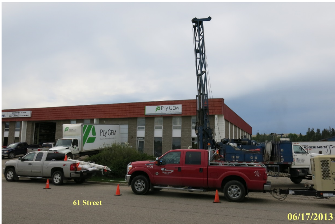
Photograph No. 6: Drilling TH-03, looking westward.
