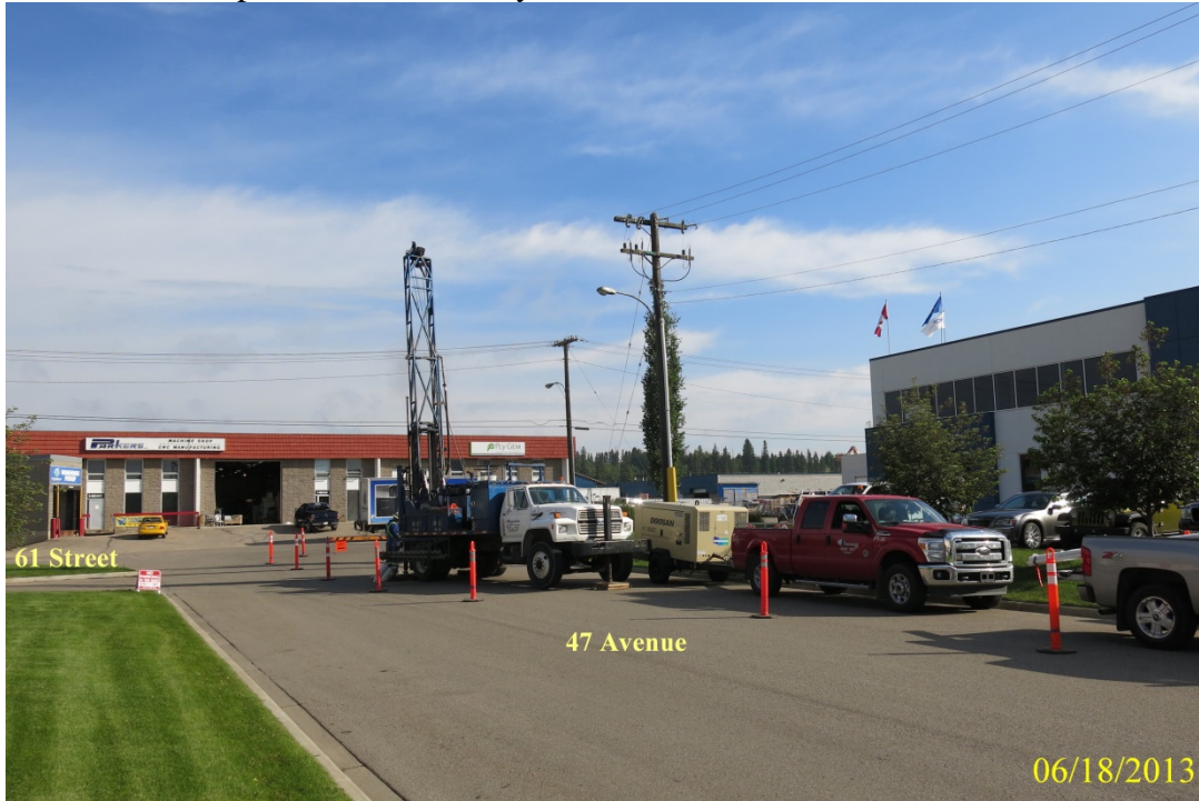
Photograph No. 5: View of set-up for drilling at MW-01.
