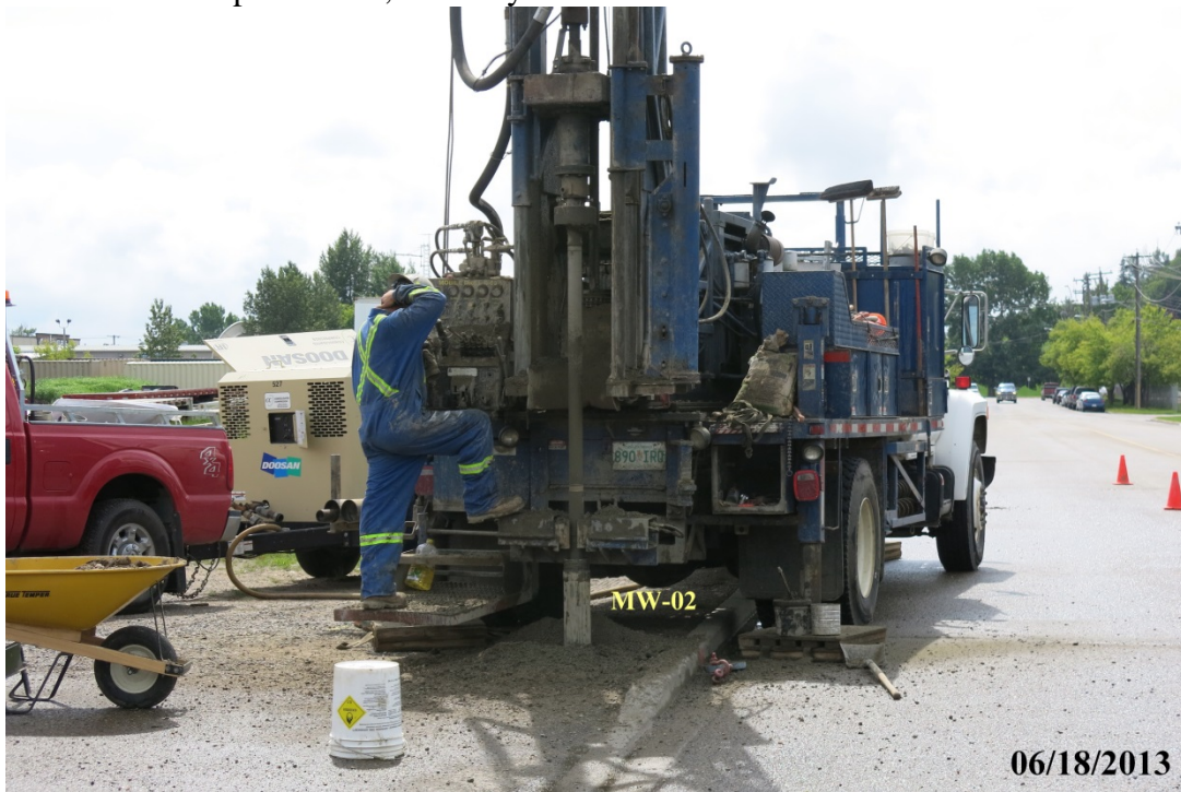
Photograph No. 7: Drilling using ODEX tooling next to 62 Street, looking southwest.
