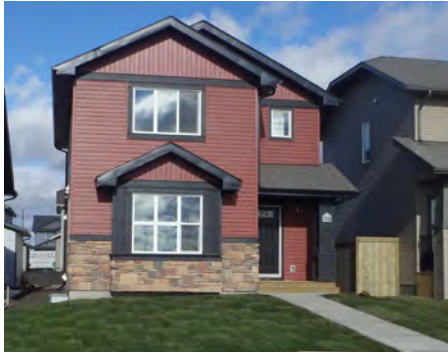
Two-storey house without front porch.
