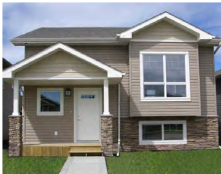
Bi-level house without front porch.
