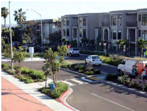
Example of bump-out traffic calming.
