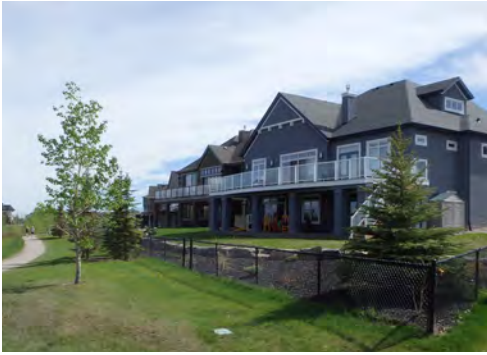
Walk-out basements with trail behind.
