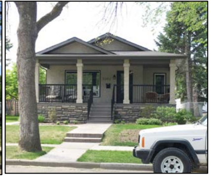
Bungalow with porch addition
