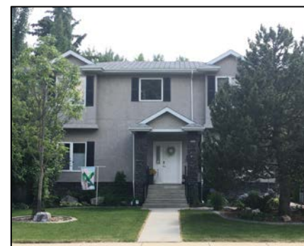
Redevelopment – second storey addition
