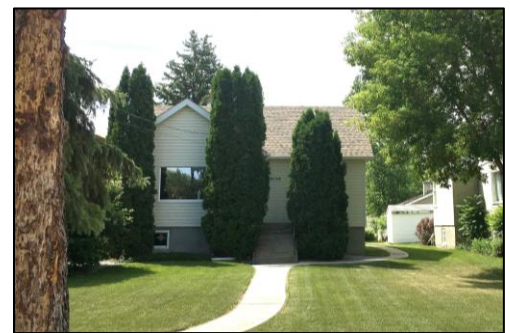
Minimal Traditional Style – renovated with vinyl siding
