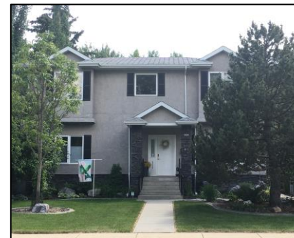
Redevelopment – second storey addition
