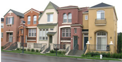
The redevelopment exception would allow medium density 2 storey housing in a single family (R1) district. Front yard setbacks of R1 would be applied to create a seamless street presence.
