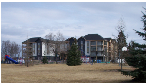
Before (top) and after (bottom) of 5601 Kerry Wood Drive. A dilapidated building was removed for construction of a condominium building.
