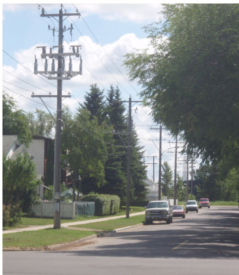
Power lines along 52 Avenue which is identified as a view corridor to the river.
