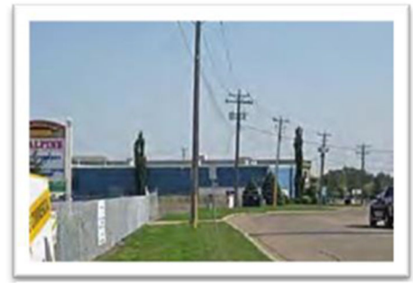
Some changes to the utility systems in Capstone will be required as redevelopment occurs
