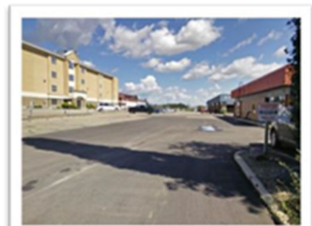
View of large parking areas within existing commercial business park area
