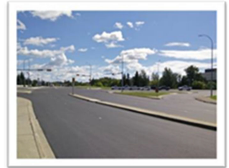
View of Taylor Drive and 45 St intersection
