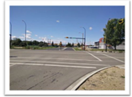
View of Taylor Drive and 47 St intersection
