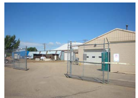
Red Deer Parks Maintenance Compound
