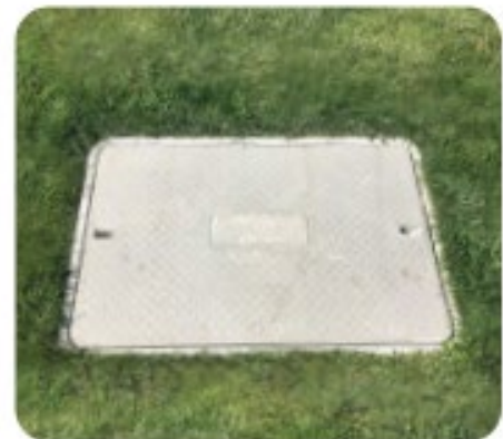
Flush-to-the-ground service boxes
