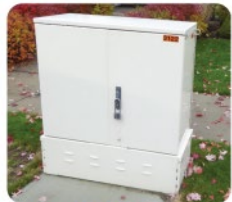
Above-ground access cabinets
