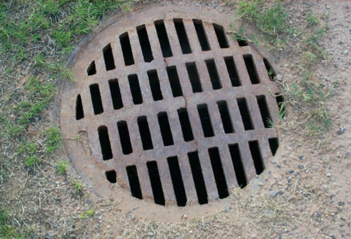
Red Deer's storm water system is designed to remove melting snow and rainfall runoff from streets and parking lots. This runoff flows directly into the river without being treated. Anything entering the storm drains, other than clean rainfall runoff, contributes to water pollution.
